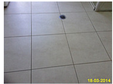
Bathroom 2/Combined with Laundry
