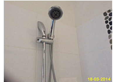
Bathroom 2/Combined with Laundry
